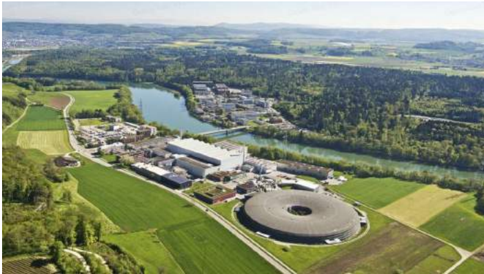
Paul Scherrer Institute in Switzerland - Cogeneration Units
